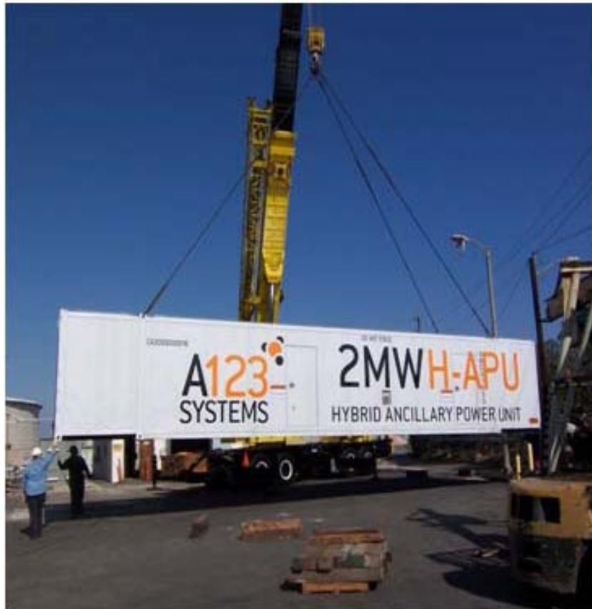
**Figure 5-10. Battery Energy Storage**
