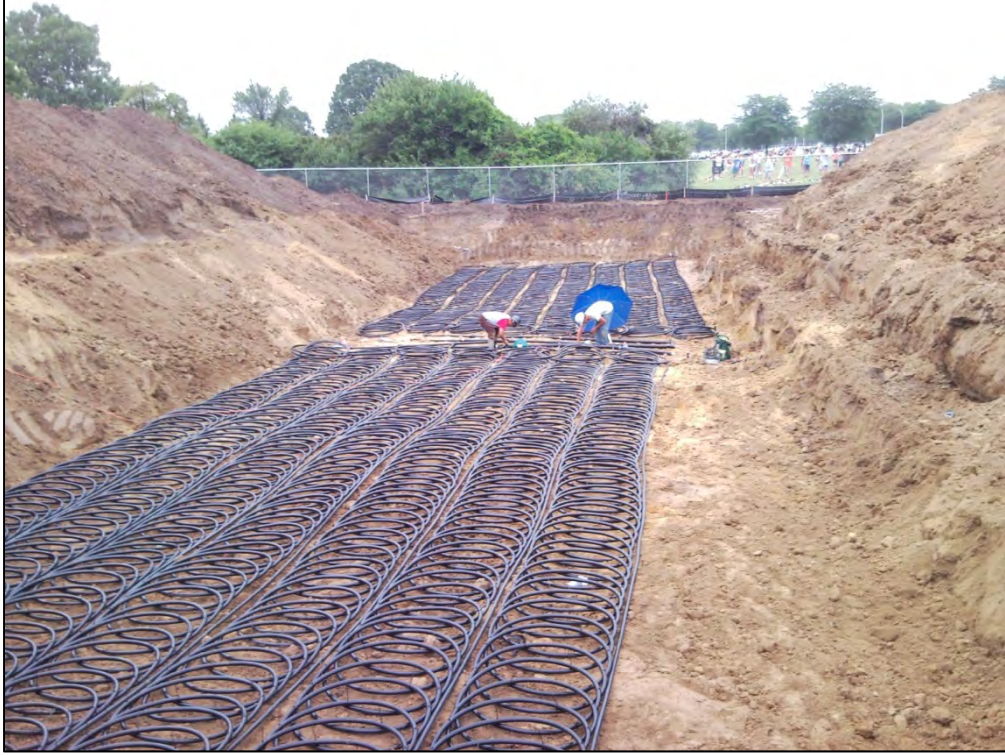
Figure 1. Geothermal Piping Installation at the Bott Building Project.
