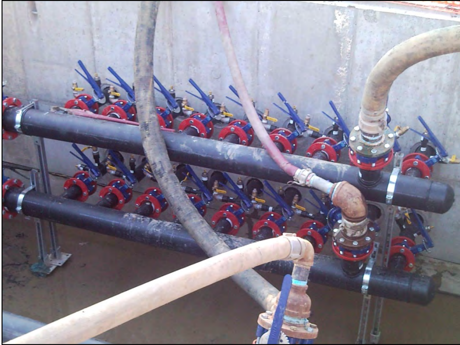
Figure 2. Header System for Geothermal Piping, Which Distributes Water to the Underground Heat Sink Loops.
