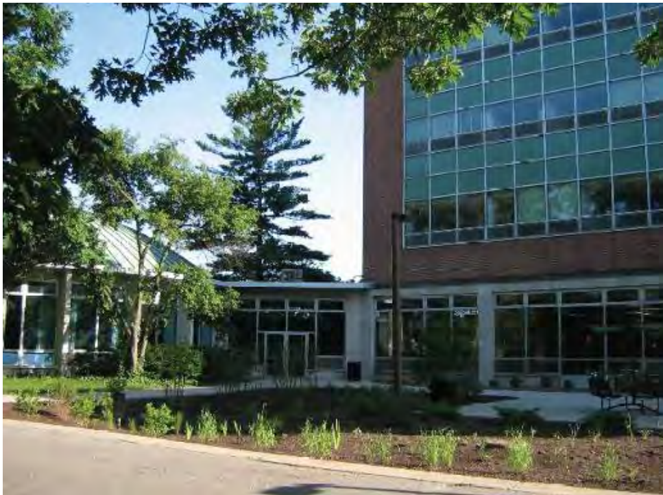
Figure 4. Erickson Hall Bioretention Basin (Rain Garden). The rain garden cleans storm water by filtering pollutants such as sidewalk salt and sediment as water drains through the soil. Cleaner water infiltrates through soil and flows into the Red Cedar River.
