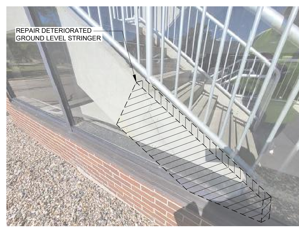
3.13 FLOOR REPAIR - STAIR STRINGER RAMP 3
