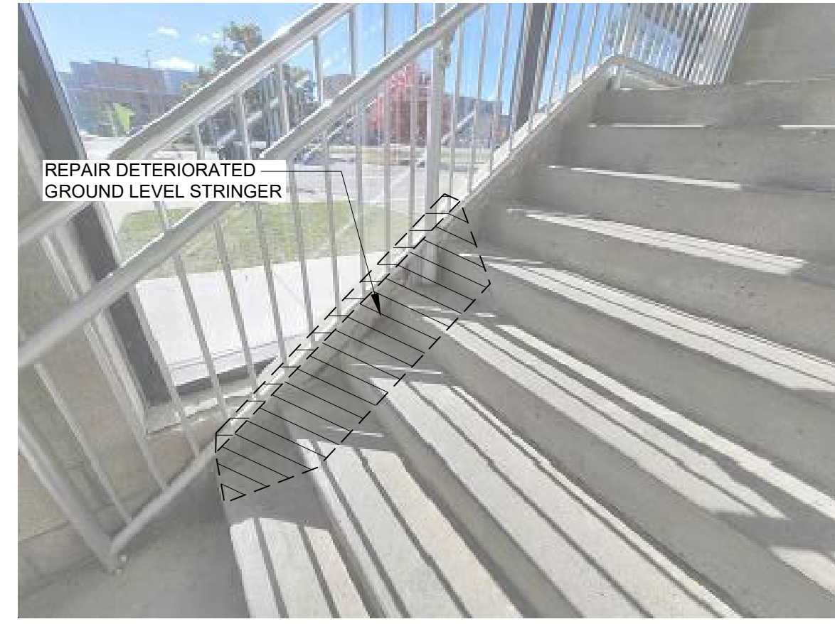
3.13 FLOOR REPAIR - STAIR STRINGER RAMP 3
