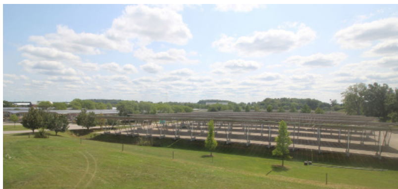
Construction progress as of August 25, 2017 on one of MSU's five commuter parking lots getting outfitted with a solar carport.
