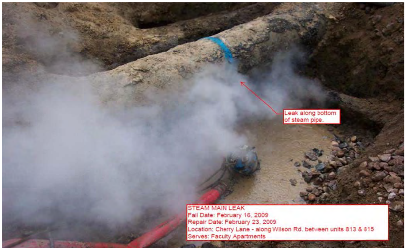
Figure 3. Direct buried steam line.
