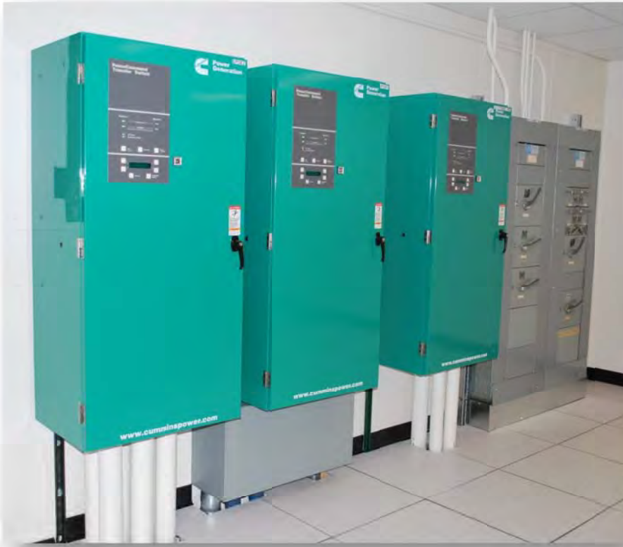
Figure 2. Data Management: Datacenters – Power Supply: Power transfer units (green boxes) enable generators to be hooked up for a manual power flip in the event of a prolonged power outage.
