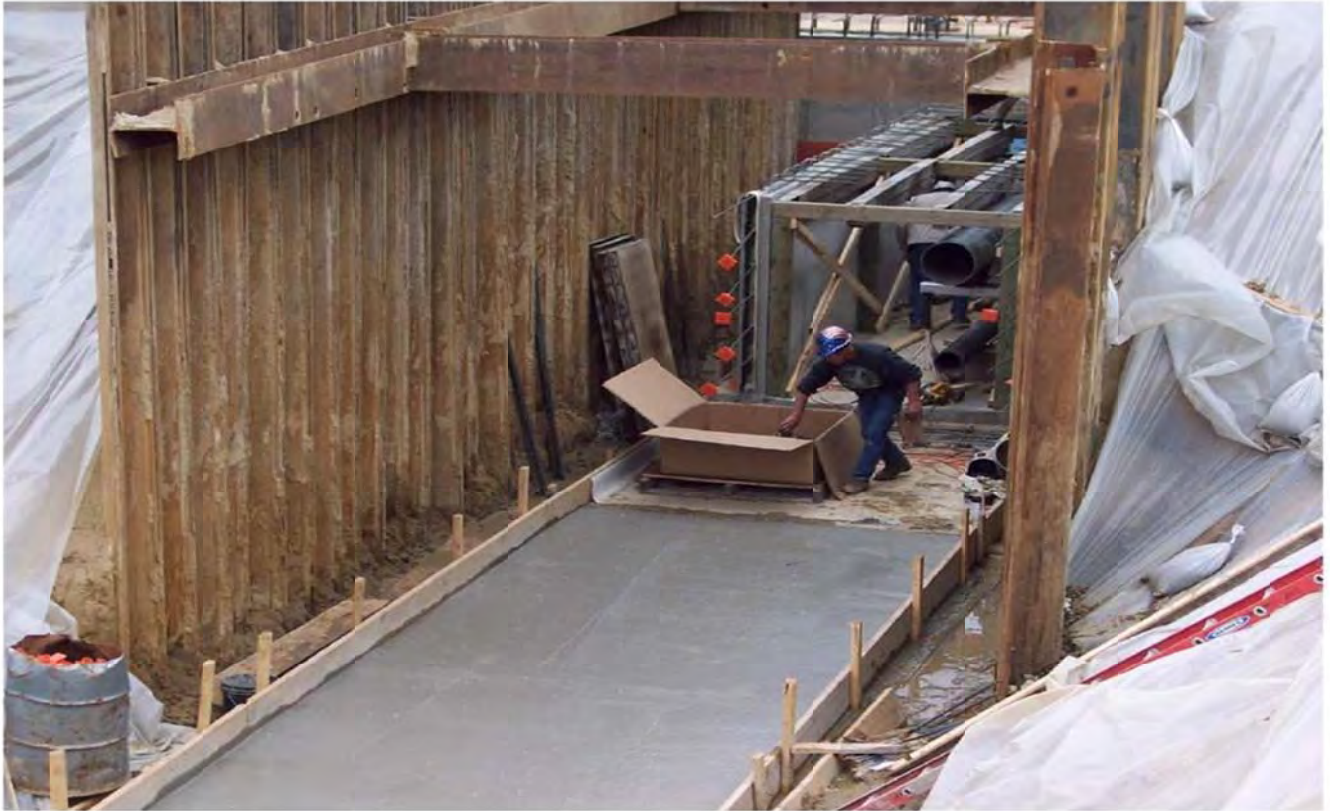
Figure 4. Steam tunnel under construction.
