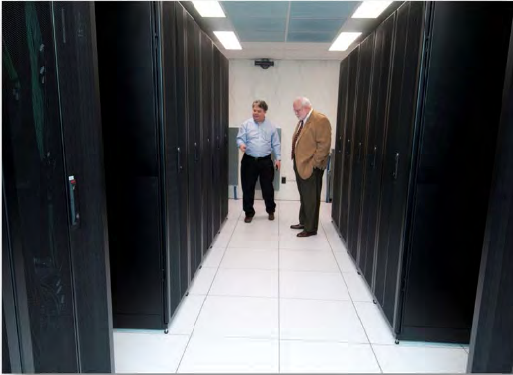
Figure 1. Data Management: Datacenters – Efficient Design: Hot and cold aisles, like in the ATS Datacenter (pictured) and the AIS Datacenter, aid in efficient energy usage.
