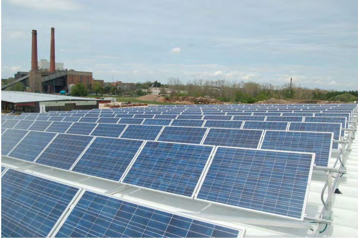
Figure 10. Photovoltaic array (solar panels) mounted on the roof of the new MSU Surplus Store and Recycling Center. The solar array generates 7-8% of the electrical needs for the new building, reducing the demand on the power plant, and is an example of how campus will move to renewable technologies T.B. Simon Power Plant is in the background.
