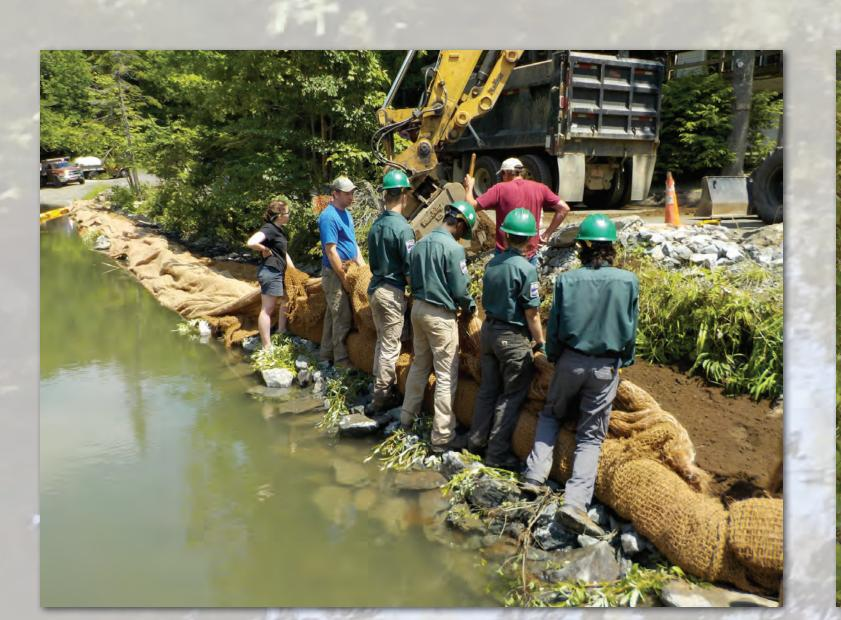
Bioengineered lift construction, using rock, coconut fiber material, soil, and native shrubs on Lake Bomoseen in Castleton, Vermont
