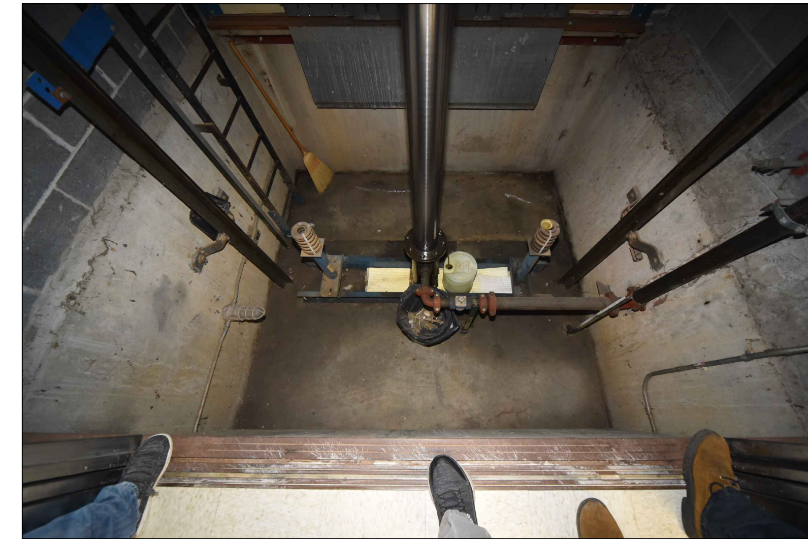
2 A5.4 EXISTING PIT, JACK, AND BUMPERS AT ELEVATOR EP4 NO SCALE
