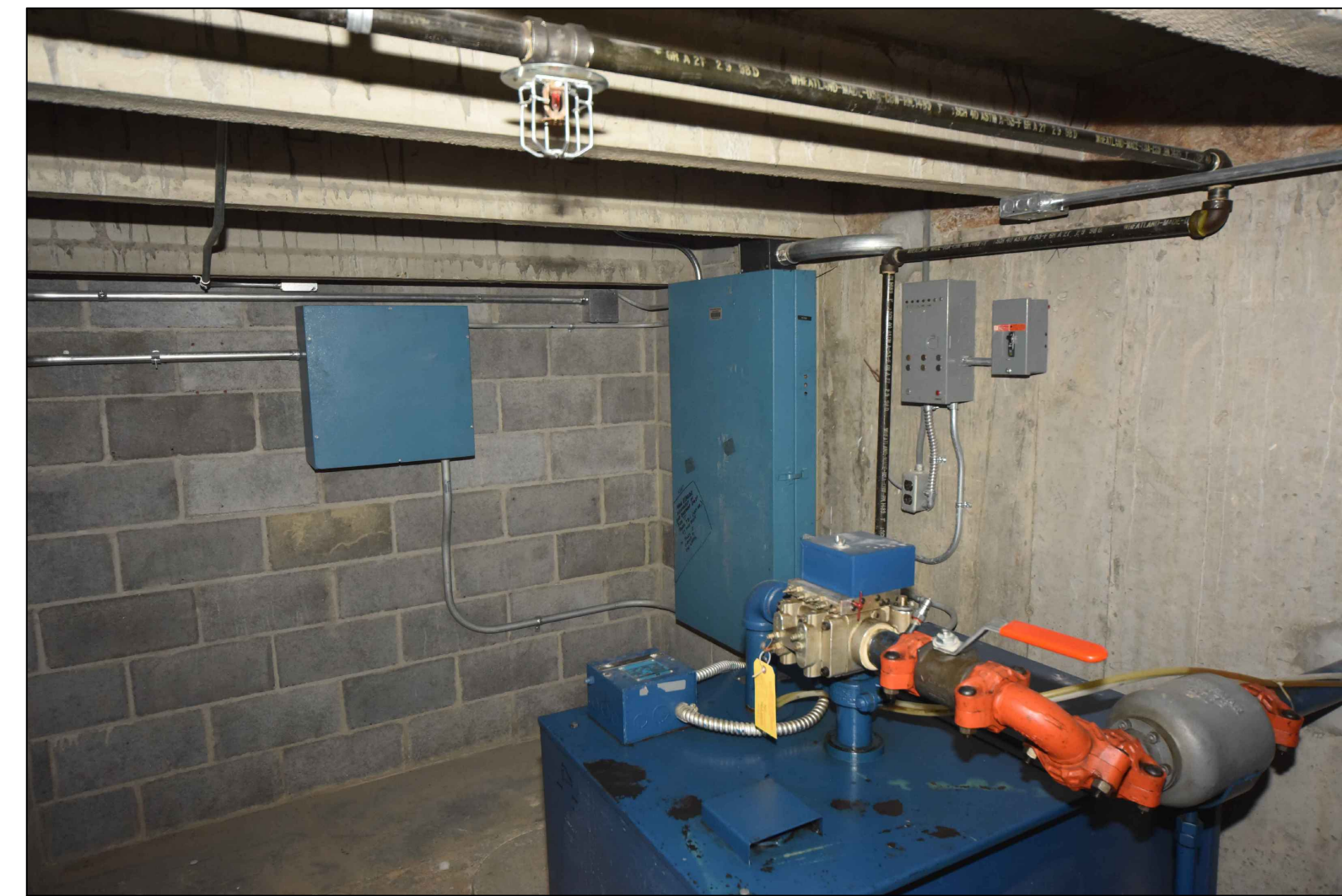
2 A5.2 EXISTING MACHINE ROOM AT ELEVATOR EP2 NO SCALE
