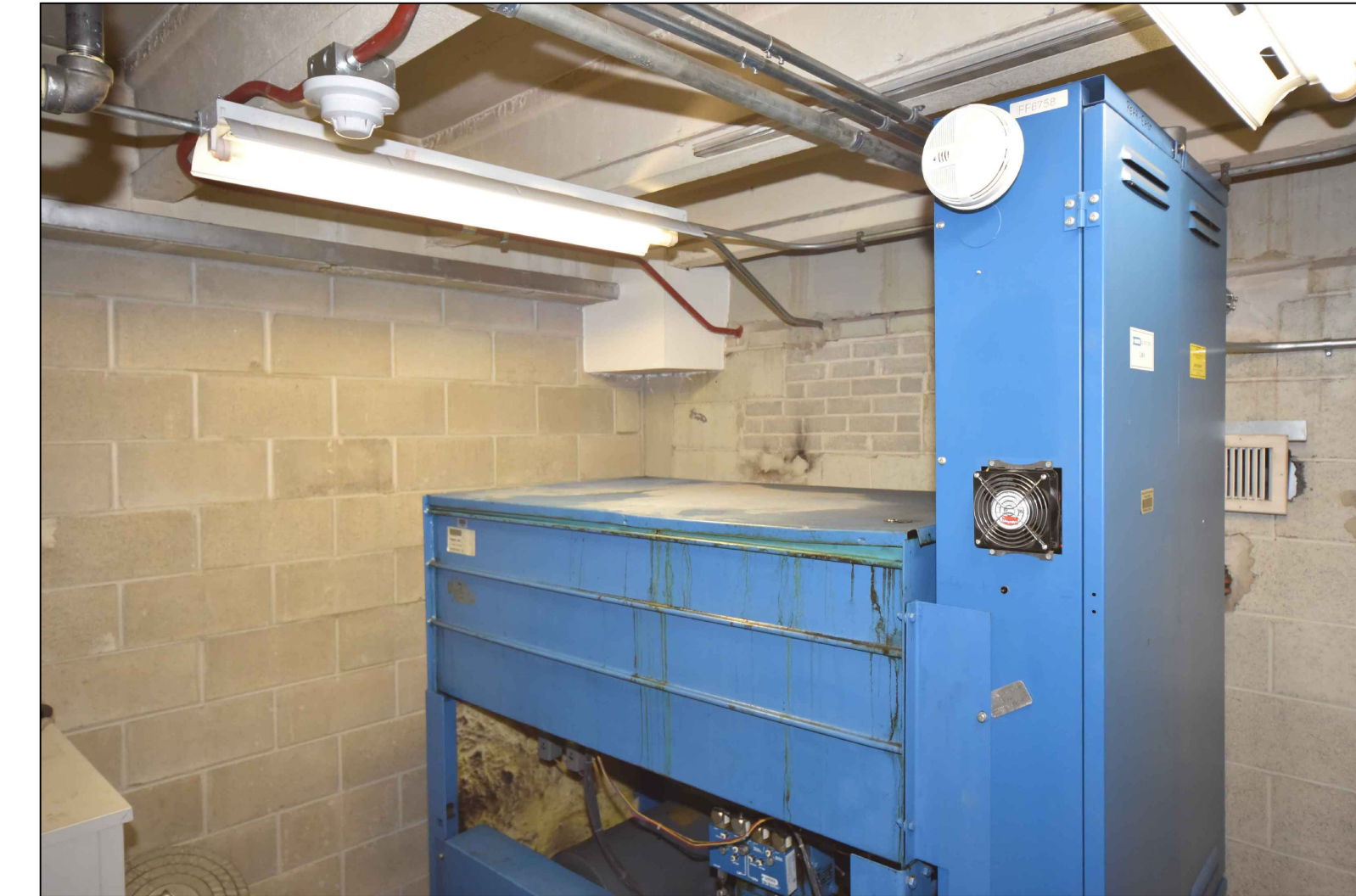
3 A5.3 EXISTING MACHINE ROOM AT ELEVATOR EP3 NO SCALE
