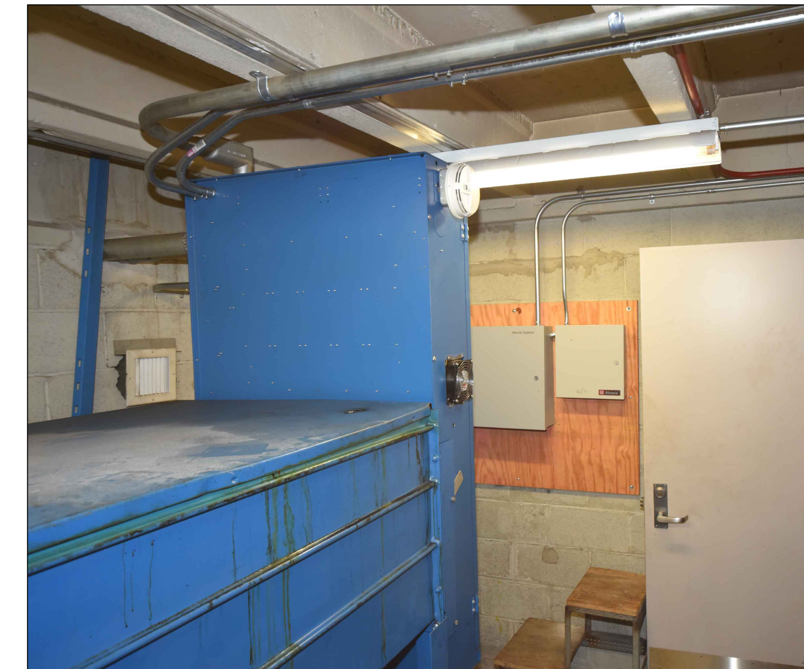
4 A5.3 EXISTING MACHINE ROOM AT ELEVATOR EP3 NO SCALE
