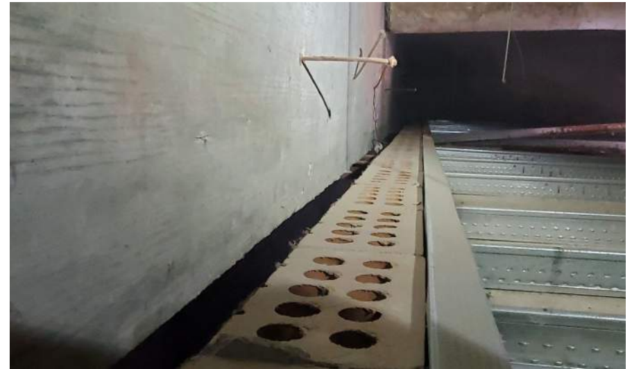
Brick walls under plaza, around louvers stop at the soffit paneling.
