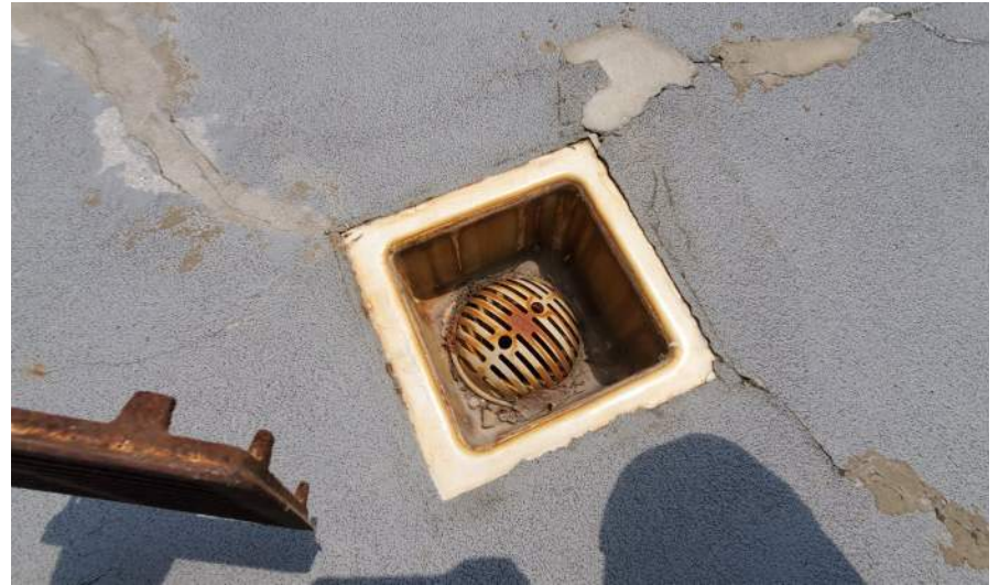
Plaza drain overview.
