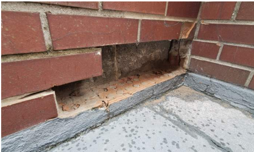
CMU back wall in sound state.
