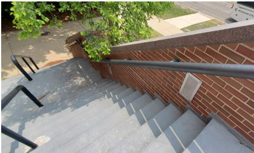
Railing used for stairway is very large and not able to fully grasp.
