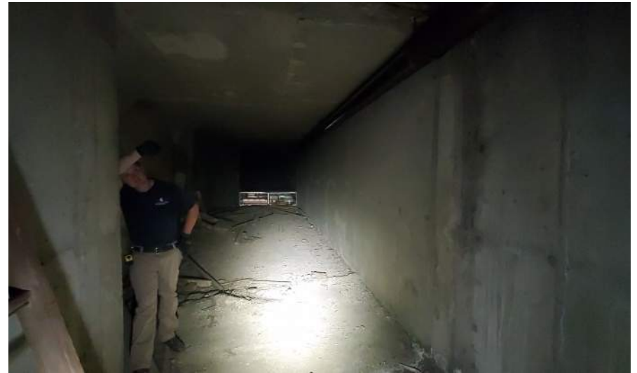
Overview of the plenum into the basement mechanical room.
