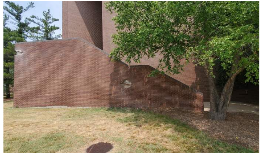
Wharton Center stair overview.
