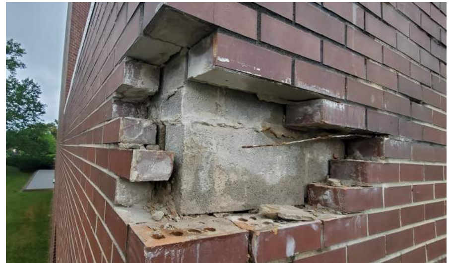
Exterior stair wall opening overview.
