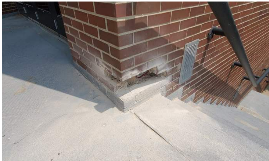
Exterior building wall opening at stairs overview.
