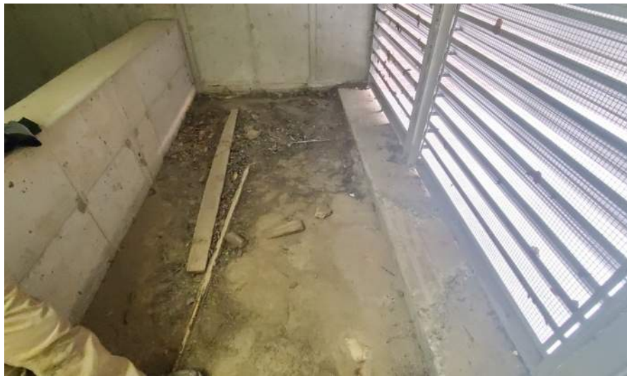
Overview of the plenum behind the exterior louver.
