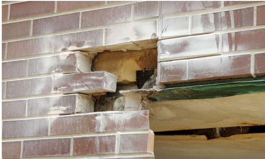
Overview where the ground level opening lintel meets Wharton Center.
