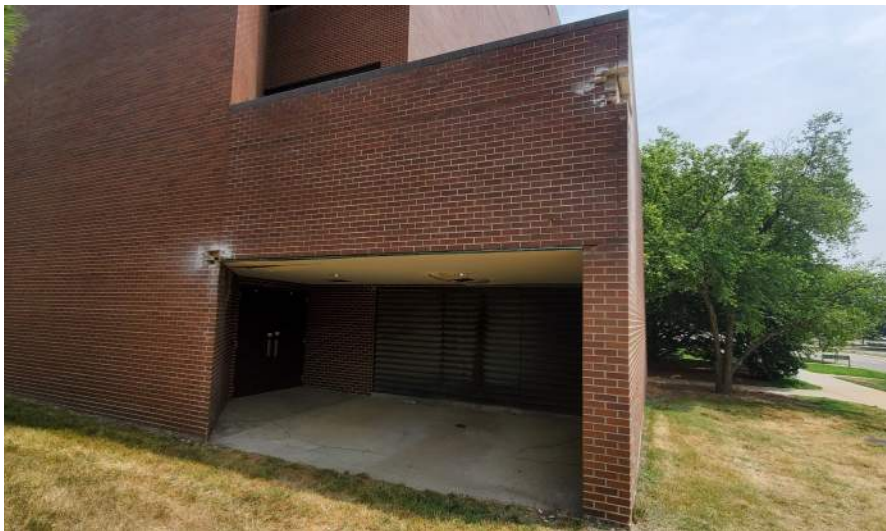
Wharton Center stair overview.
