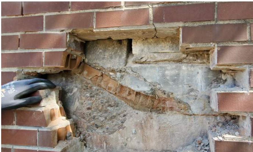
Exterior stair wall opening overview.
