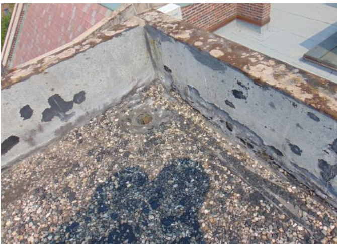
Photo 23: Area 7 - deteriorated surface and base flashing
