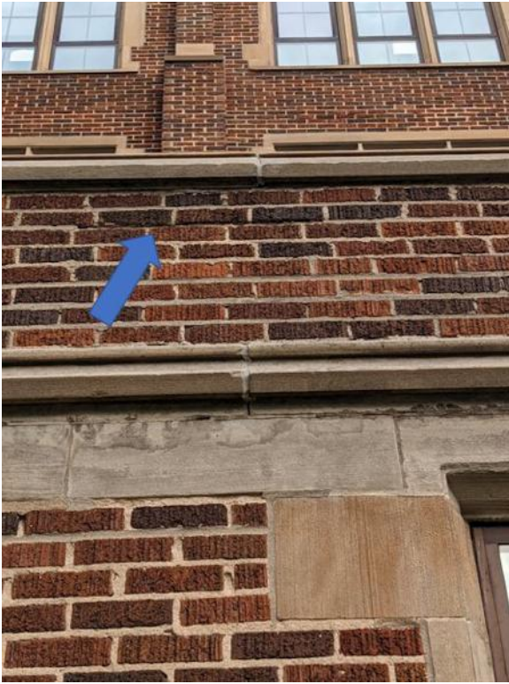
Photo 13: Typical eroded mortar joints
