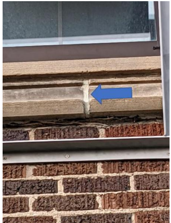
Photo 4: Typical head joint to be caulked
