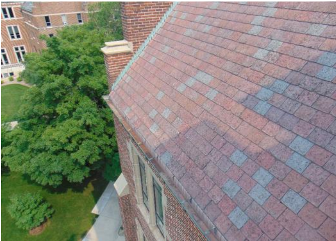
Photo 9: Area 1 - stained/weathered asbestos tiles
