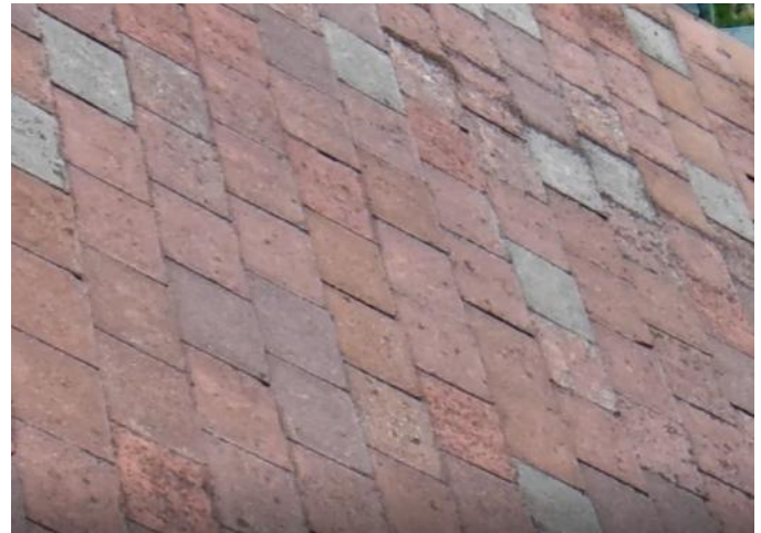
Photo 16: Area 5 - stained/weathered/broken asbestos tiles
