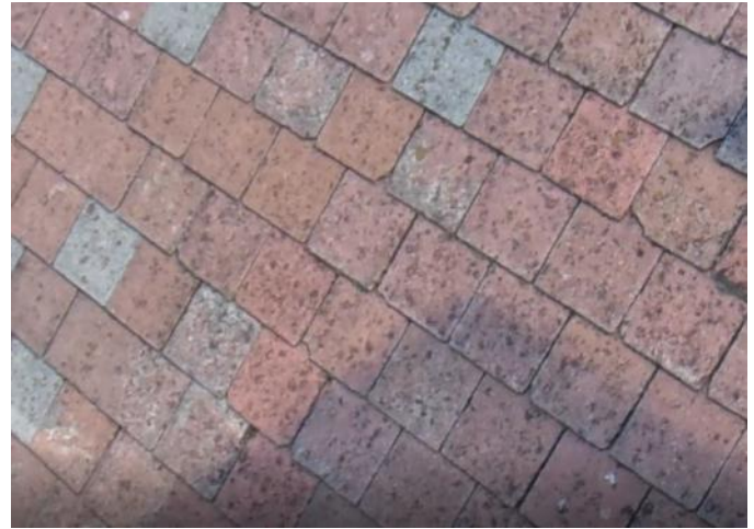
Photo 8: Area 1 - stained/weathered/broken asbestos tiles
