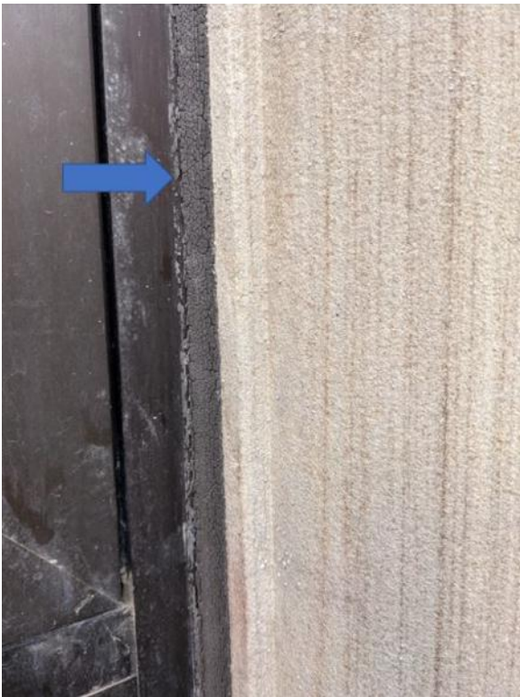
Photo 1: Typical defective caulking around the perimeter of windows
