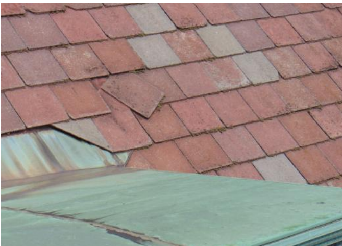
Photo 35: Area 11 - loose/broken asbestos tiles
