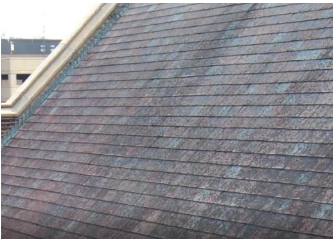
Photo 17: Area 5 - west facing - stained/weathered/broken asbestos tiles
