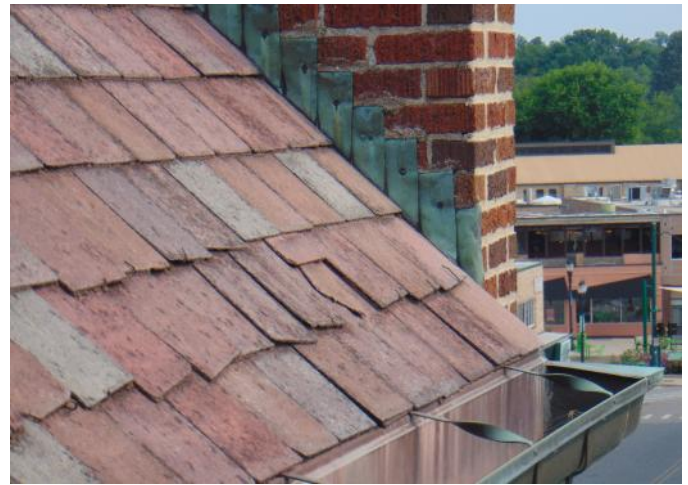
Photo 14: Area 5 - stained/weathered/broken asbestos tiles
