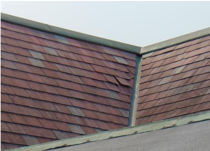
Photo 39: Area 11 - loose/missing asbestos tiles
