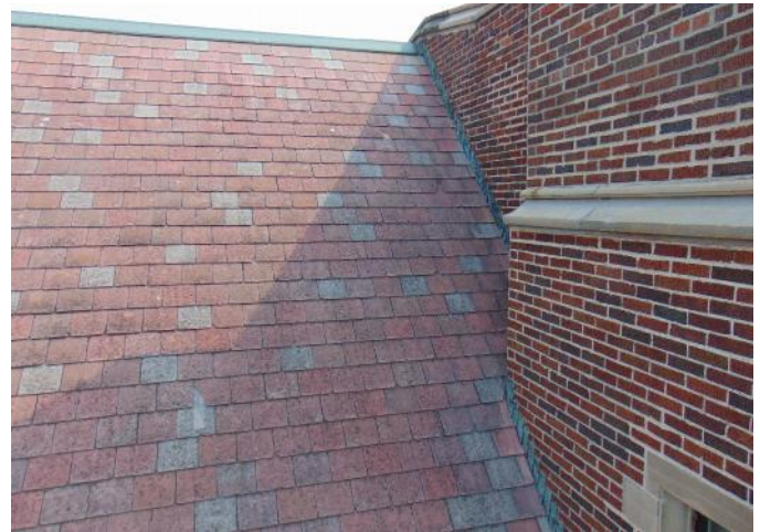
Photo 10: Area 1 - stained/weathered asbestos tiles
