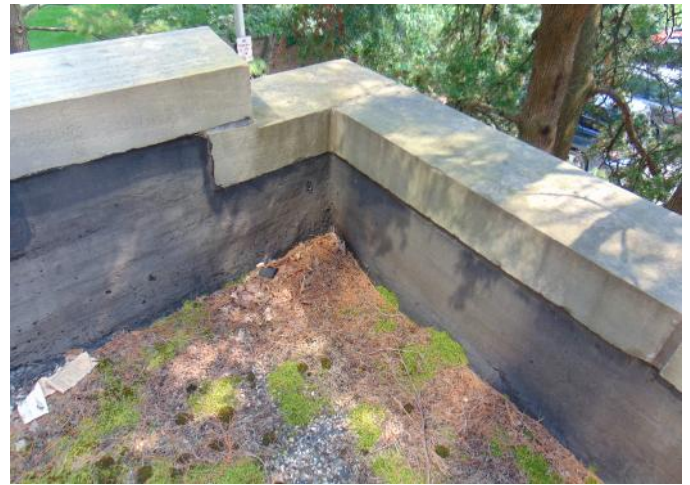
Photo 14: Area 4 - debris/vegetation - base flashing surface wear
