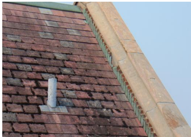
Photo 2: Area 1 - stained/weathered/moss growth between asbestos tiles
