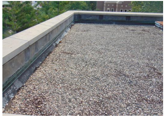
Photo 8: Area 3 - deteriorated base flashing
