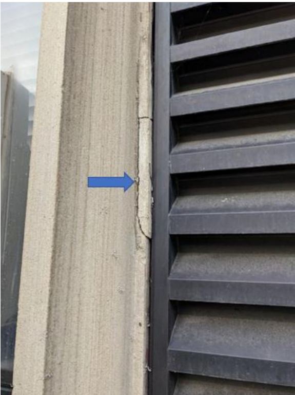
Photo 15: Typical stone patching
