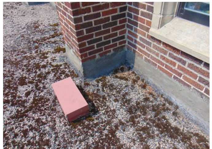
Photo 12 Area 4 -debris/vegetation - base flashing surface wear
