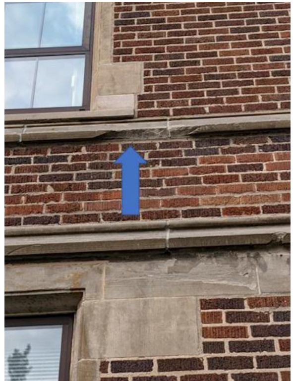
Photo 16: Typical stone patching
