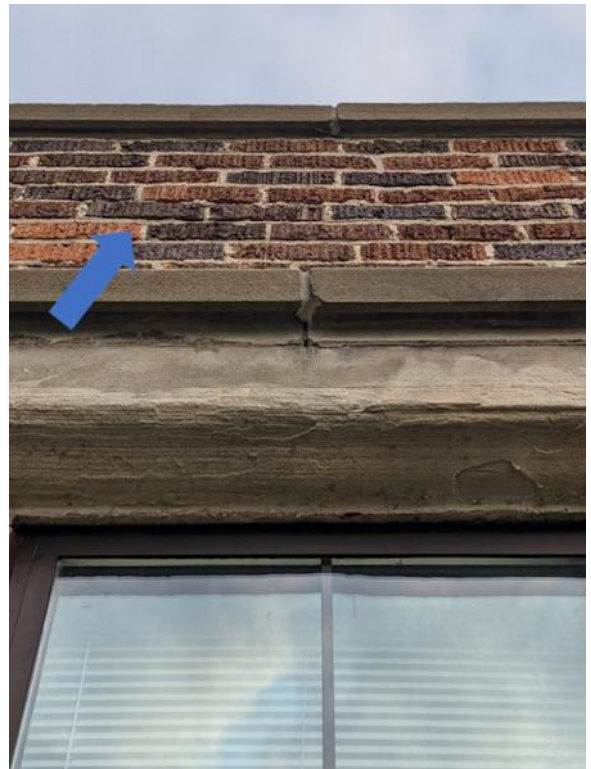
Photo 12: Typical eroded mortar joints
