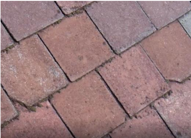
Photo 15: Area 5 - stained/weathered/broken asbestos tiles
