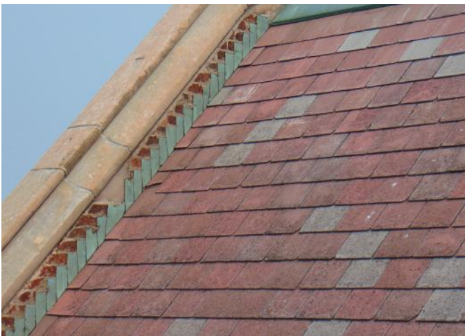
Photo 11: Area 1 - stained/weathered/broken asbestos tiles
