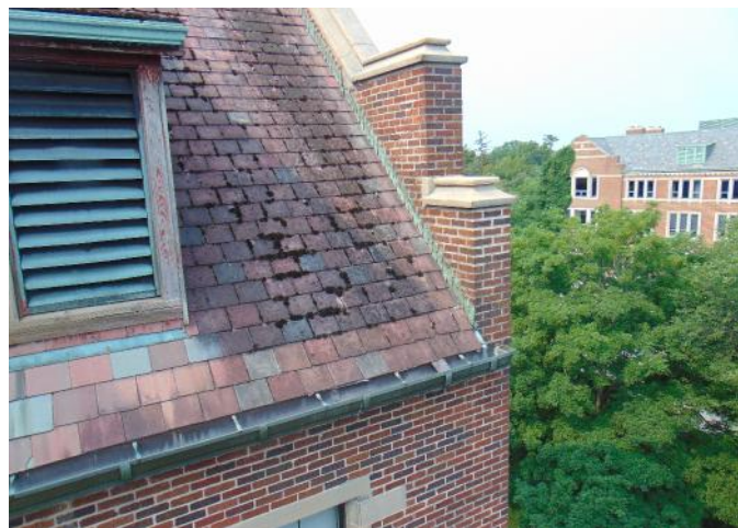
Photo 4: Area 1 - stained/weathered/moss growth between asbestos tiles
