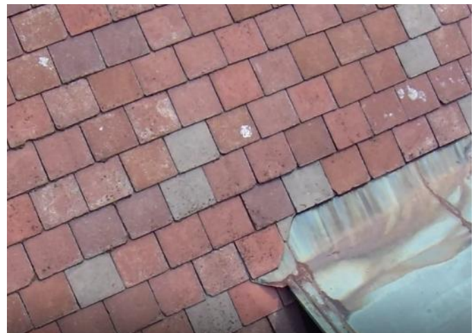
Photo 30: Area 11 - stained/weathered/broken asbestos tiles
