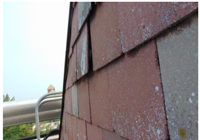
Photo 42: Area 11 - north facing - loose tiles on dormer wall
