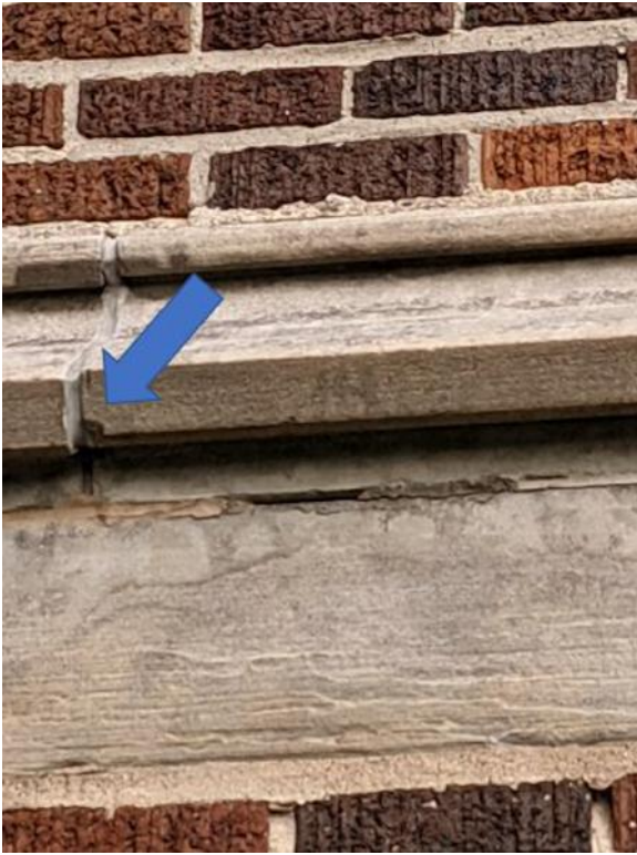
Photo 5: Typical head joint
