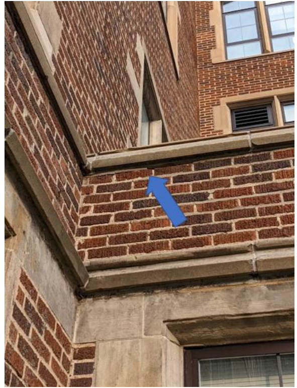
Photo 14: Typical eroded mortar joints
