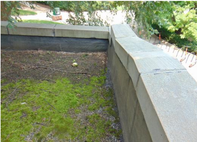
Photo 3: Area 2 - debris/vegetation accumulation in corner
