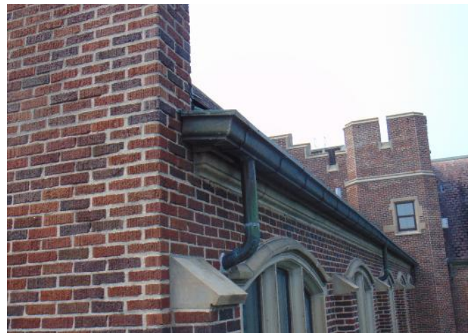
Photo 24: Area 5 - gutter and downspouts
