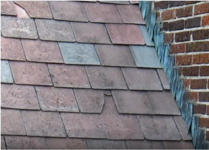
Photo 7: Area 1 - broken asbestos tiles - bent step flashing
