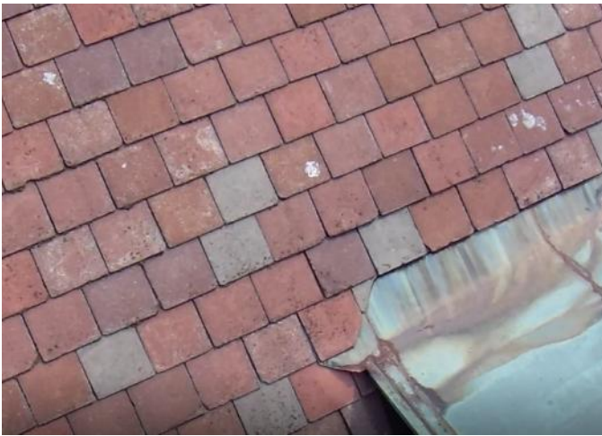
Photo 31: Area 11 - stained/weathered/broken asbestos tiles
