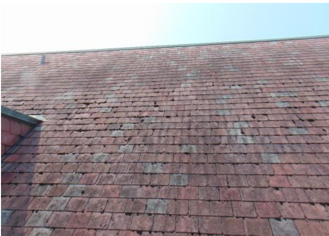
Photo 41: Area 11 - moss growing between asbestos tiles
