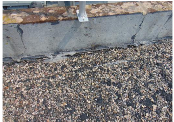
Photo 22: Area 7 - deteriorated surface and base flashing
