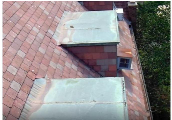
Photo 28: Area 11 - stained/pitting copper on dormer cap roofs
