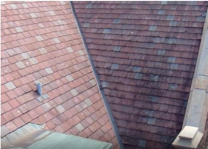
Photo 27: Area 11 - stained/weathered/broken asbestos tiles
