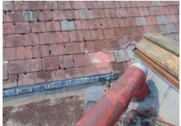
Photo 40: Area 11 - north facing - moss growing between asbestos tiles
