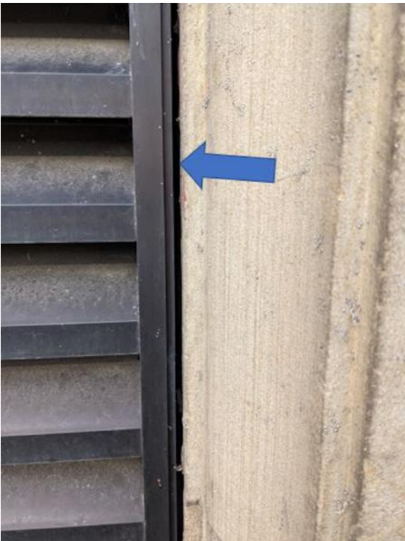
Photo 3: Missing caulking around louver
