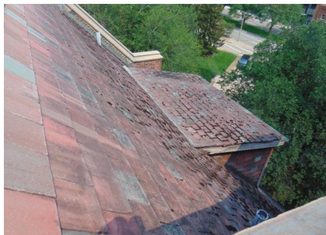
Photo 6: Area 1 - slope of dormer roof is inadequate to provide required drainage of a tile
