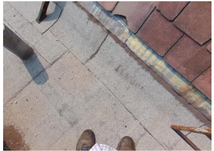
Photo 26: Area 8 - membrane in good condition
