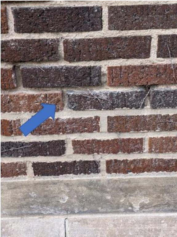
Photo 9: Typical eroded mortar joints
