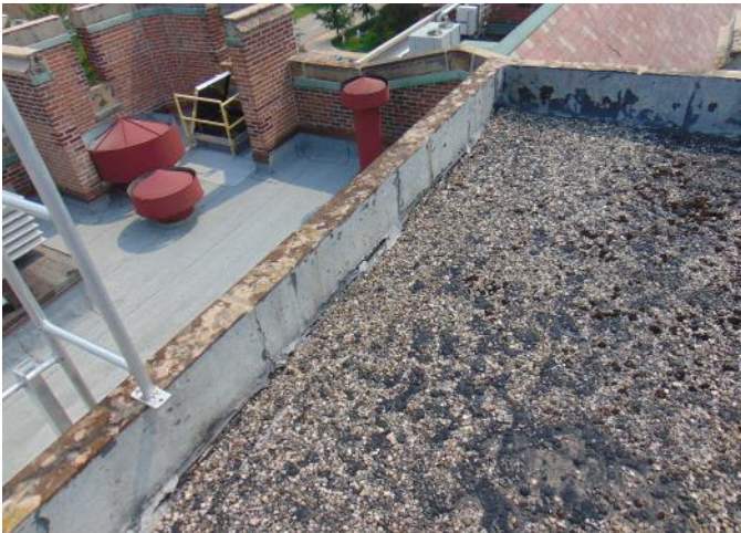
Photo 21: Area 7 - deteriorated surface and base flashing
