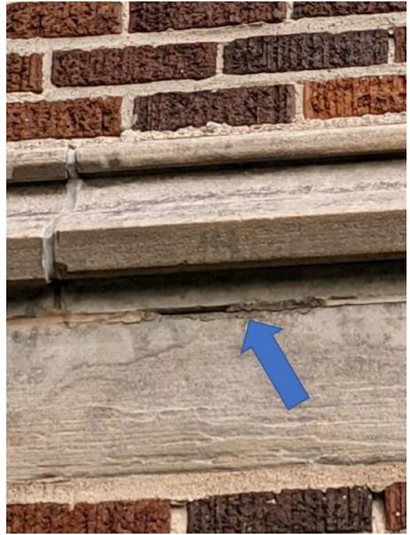
Photo 6: Typical deteriorated mortar joint
