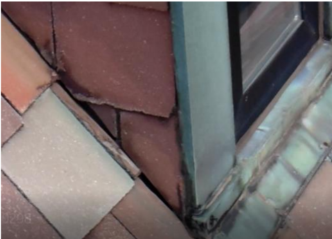
Photo 33: Area 11 - stained/pitted copper trim at dormer windows
