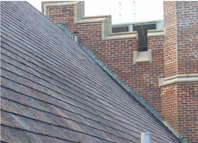
Photo 21: Area 5 - stained/weathered/broken asbestos tiles
