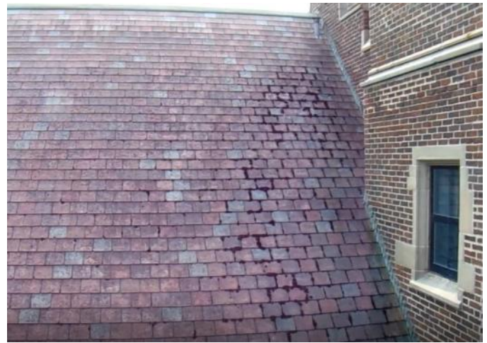
Photo 20: Area 5 - stained/weathered/moss growing between asbestos tiles
