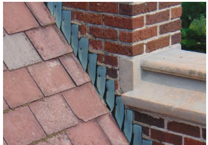
Photo 36: Area 11 - stained/weathered/broken asbestos tiles - bent step flashing
