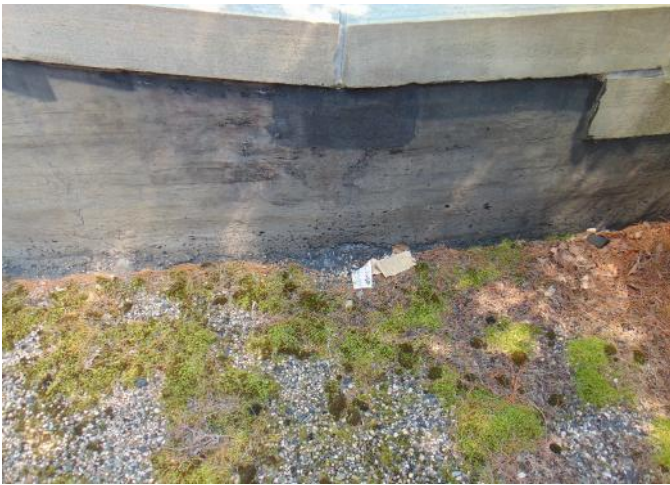
Photo 13: Area 4 - debris/vegetation - base flashing surface wear
