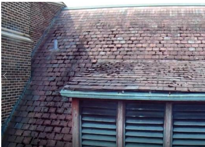
Photo 1: Area 1 - stained/weathered/moss growth between asbestos tiles
