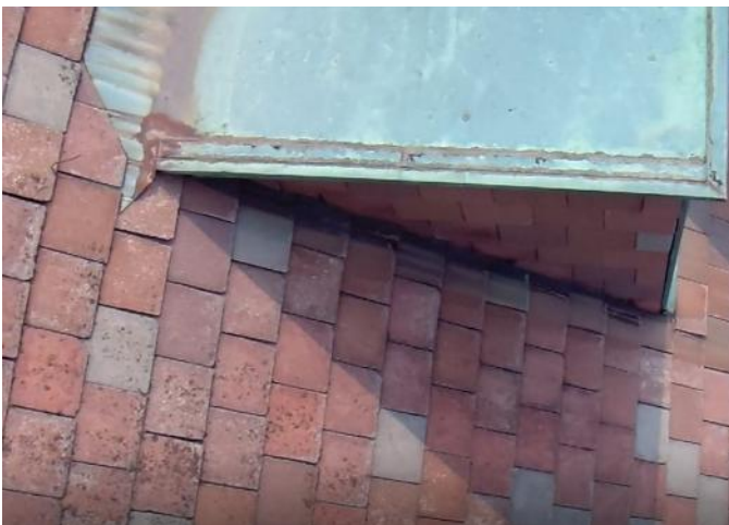
Photo 29: Area 11 - stained/pitting copper on dormer cap roofs
