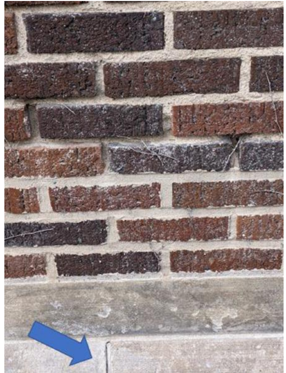
Photo 10: Typical head joint
