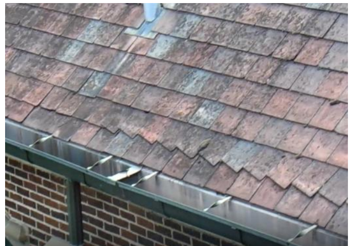
Photo 18: Area 5 -stained/weathered/broken asbestos tiles
