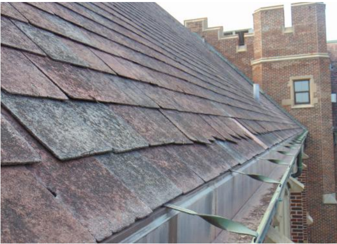
Photo 19: Area 5 - stained/weathered/broken asbestos tiles
