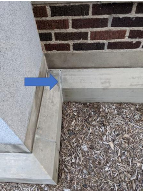
Photo 7: Typical head joint
