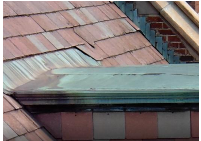
Photo 34: Area 11 - stained/weathered/broken asbestos tiles - stained/pitted copper
