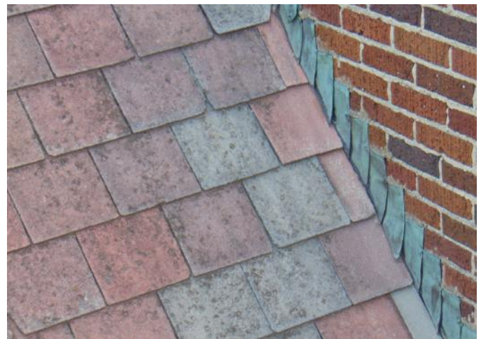
Photo 12: Area 1 - stained/weathered/broken asbestos tiles - bent step flashing
