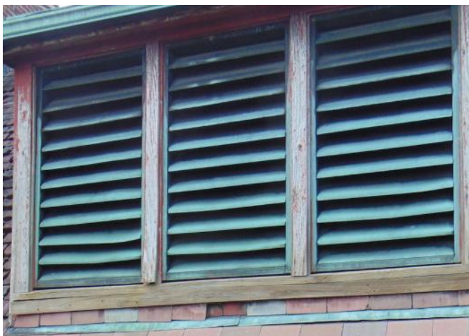
Photo 3: Area 1 - weathered lumber around louvers - missing asbestos tiles
