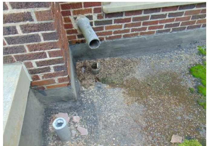
Photo 6: Area 2 -broken drain strainer
