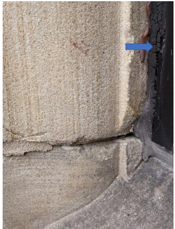
Photo 2: Typical defective caulking around the perimeter of windows
