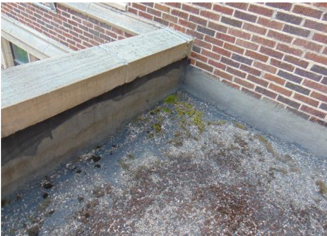
Photo 15: Area 4 - debris/vegetation - base flashing surface wear
