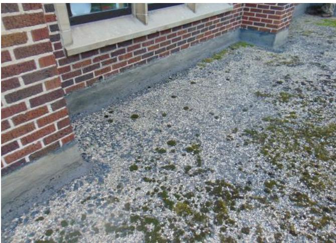
Photo 5: Area 2 -base flashing surface wear
