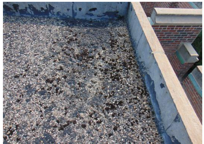
Photo 24: Area 7 - deteriorated surface and base flashing
