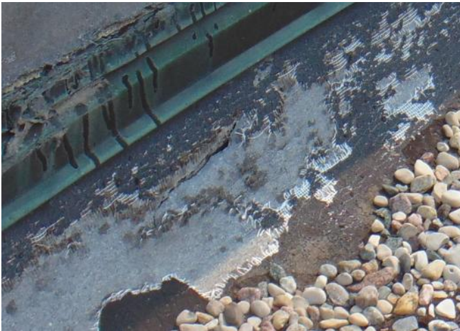
Photo 9: Area 3 - deteriorated base flashing
