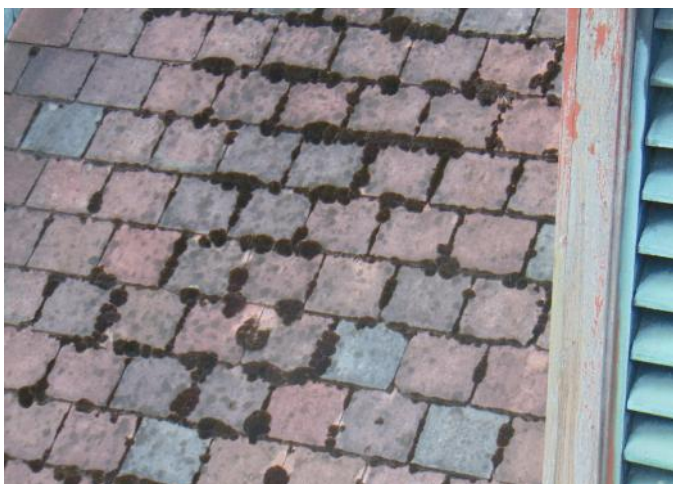
Photo 5: Area 1 - stained/weathered/moss growth between asbestos tiles
