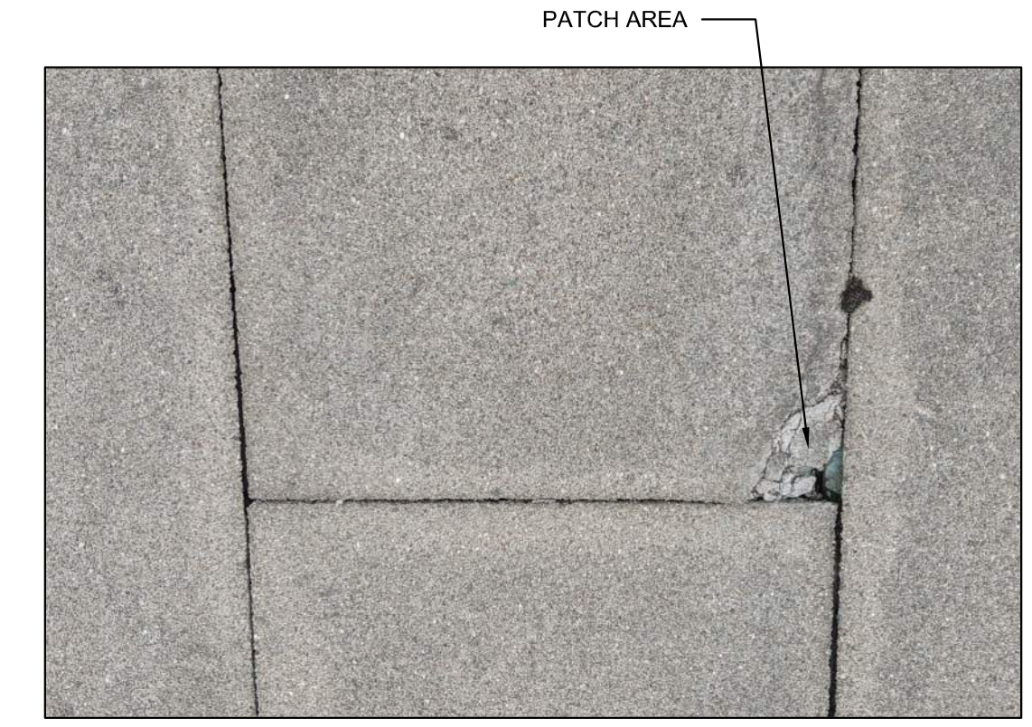
REINSTALL SAWCUT PARTIAL PANEL PANEL CAN BE RE-INSTALLED FOLLOWING PATCH AND REPAIR; REFER TO TECH NOTE IN PROJECT MANUAL
